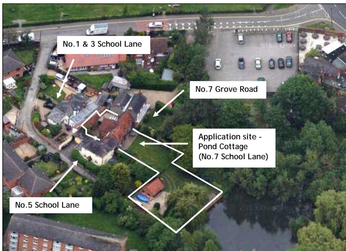
Figure 1.2 - Aerial view of application site from the south
