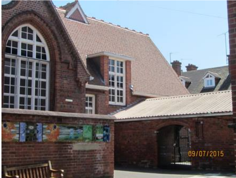
Rear elevation of canopy with existing access
