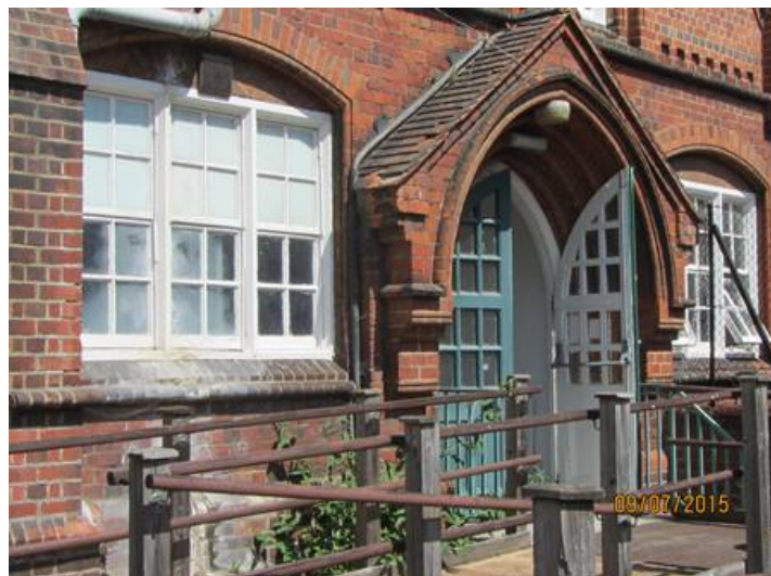
Original entrance door with ramp
