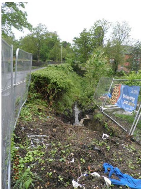
View west along rear of dam embankment from within allotment site
