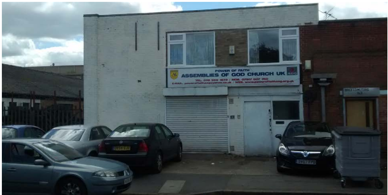
Site photograph showing the front elevation of the building (03/06/2015)
