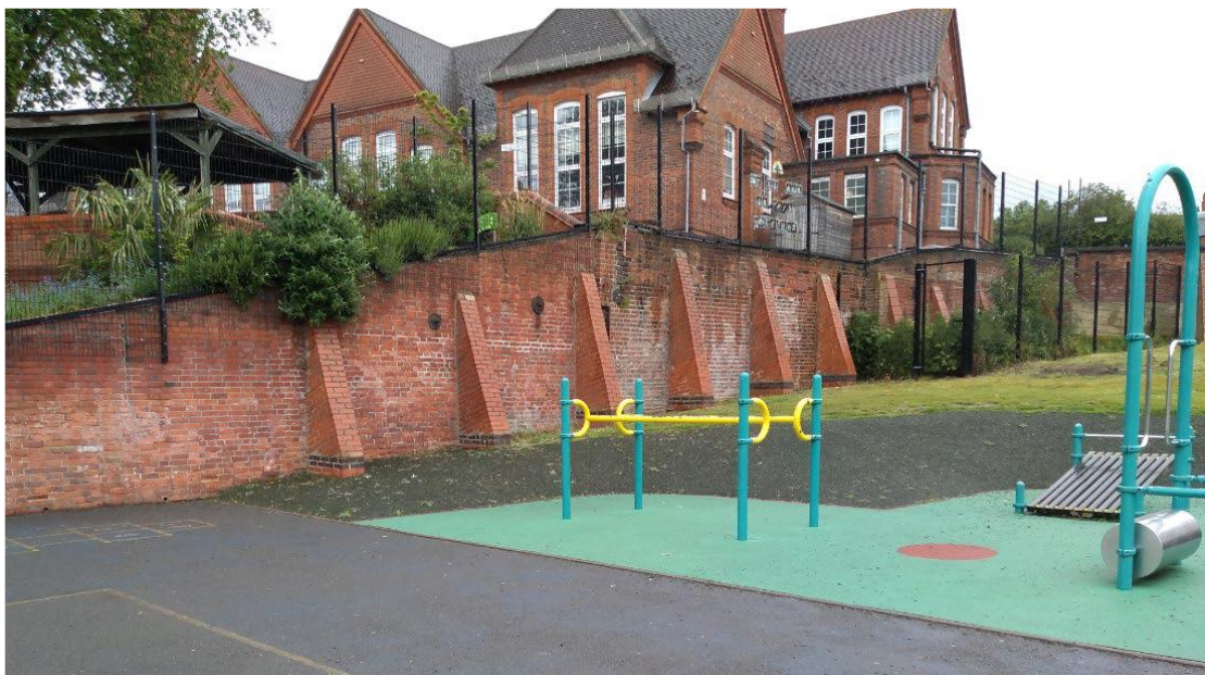
South-facing elevation showing modern buttresses
