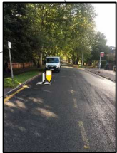
PROPOSED RUBBER KERBING WITH TMP BOLLARDS AND TAPER ACTING AS TRAFFIC CALMING FEATURES
