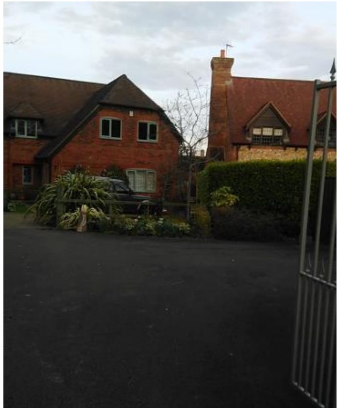
Looking towards No 7 on the left and No 8 on the right
