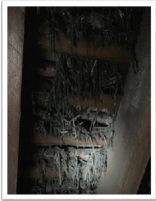
Photo 5 & 6: Remains of possible straw and plaster torching below tiles where roof voids accessible.
