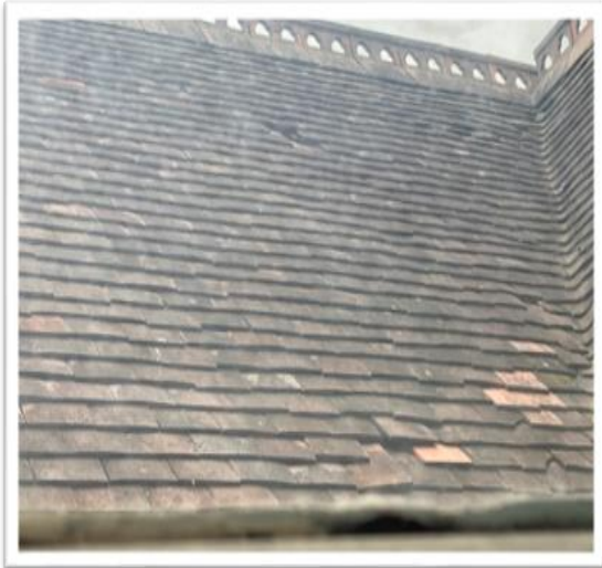
Photo 3 & 4: Existing roof section showing slipped/missing tiles & recent replacements
