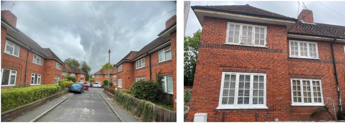
Figures 1 and 2. View of Barry Place and a Semi with original fenestration on Barry Place
