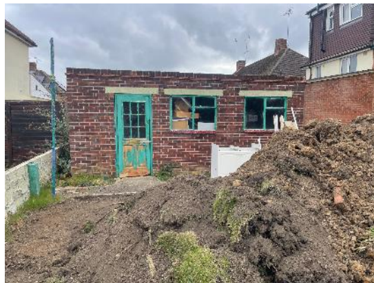
Figure 3. Image of the garage
