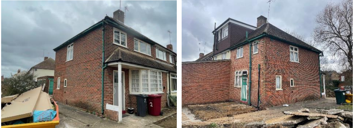
Figures 1 and 2. Image of the front, side and rear elevations of the property
