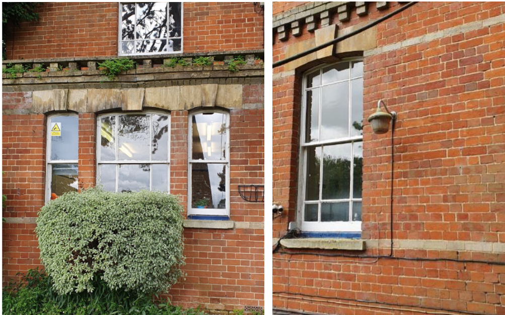
Figures 2 and 3. Details of brick bonding: Flemish bond on the principal façade (left), the mixture of Flemish and English Bond on the southern façade (right) (photographs are from an appendix of the nomination file)
