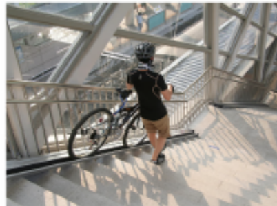
staircase to accommodate cycle rail
