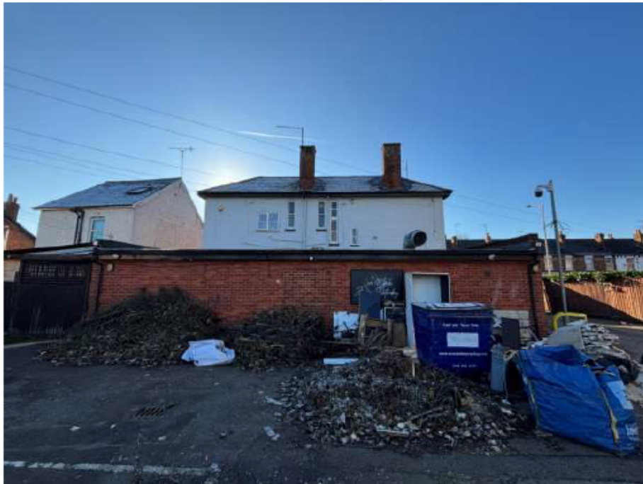
Figure 24: The rear elevation of the subject site showing the substantial 1970s single storey rear extension.
