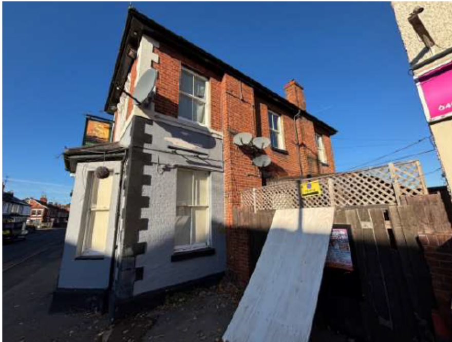
Figure 23: View of the eastern (side) elevation showing the lean-to shelter to the side of the building and the previously removed chimney stack.
