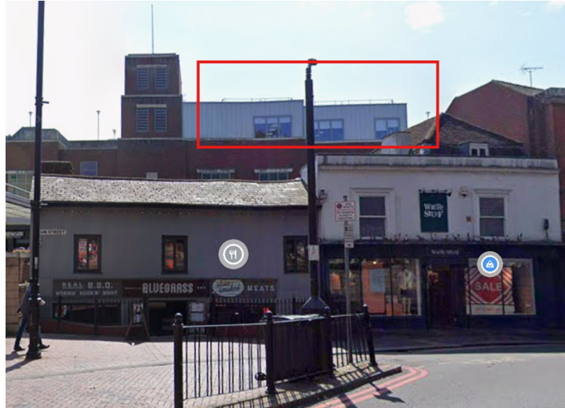
Figure 15– view of existing safety rails to roof of The Oracle looking south from Gun Street
