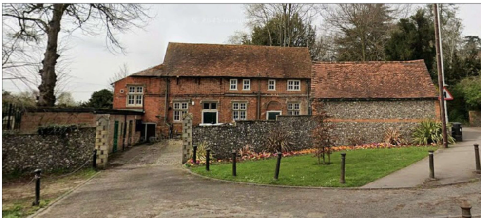
01 Stable Block Gateway & Piers from Highway NTS
