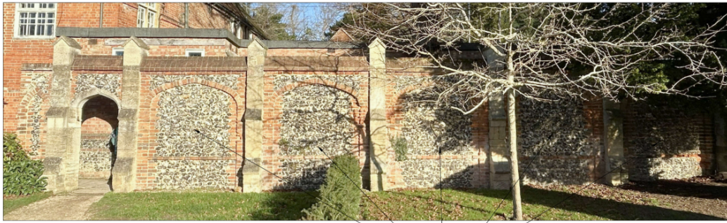
01 Boundary Wall - Caversham Court Gardens NTS
